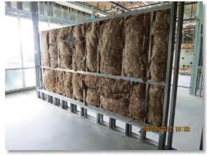
Have a pre-installation meeting to allow for proper planning of the entire system, including studs, mechanical, electrical, insulation, sound attenuation on boxes, installation sequencing, <u>verification</u>, and final attachment coordination.
