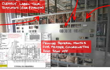
Build metal stud framing into head wall assembly – coordinate the stud locations with millwork, access, installation, etc.
