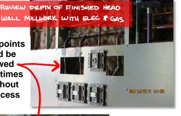
An installation of a header at top & bottom will allow for the room framing to continue aheadof the head wall installation.
